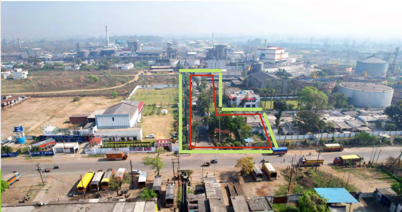
DB GATE TO RDL MAIN GATE & COLONY AREA PLANTS 395 NOS
